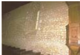
126. Dragey. The north wall of the nave (inside). Villagers patiently scraped the plaster to show the opus spicatum (fishbone masonry), a sign their church was early Romanesque. The inner plaster now only covers the last top quarter of the walls, probably too hard to reach. Photo by Claude Rayon. [Claude_37]
