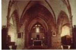
146. Genêts. The Romanesque transept crossing is bounded by four strong square piers. The two west piers are attached to the transept and the nave. They receive four thick triangular arches that surround the groin vault above the transept crossing. The first row of the choir opens north and south on two flat apse chapels, that open themselves on the transept arms. Photo by Alain Dermigny. [Alain_078]
