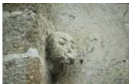
029. Bréville. Above the Romanesque gate in the south base of the tower, a human head carved in a limestone didn't resist well to the test of time, unlike the heads carved in granite in the south gate of the church of Yquelon. Photo by Alain Dermigny. [Alain_013]
